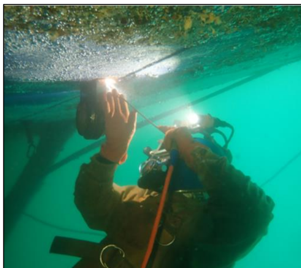
Fig.1. Work of underwater welding technology
